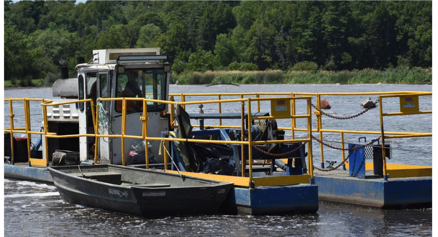
The desludging is a critical component of operations underway to minimize odours coming from the primary lagoon at the plant. This work is slated to continue into mid-August.
